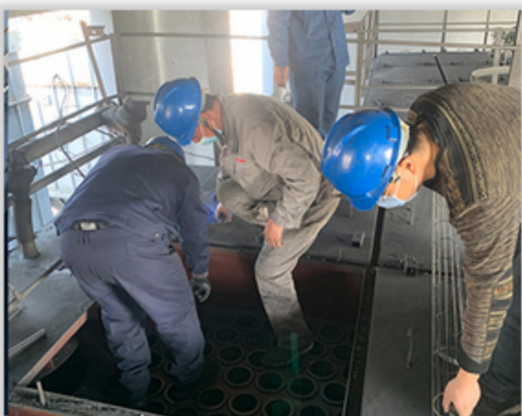
install Pleated Bag Cartridges in Carbon plant
