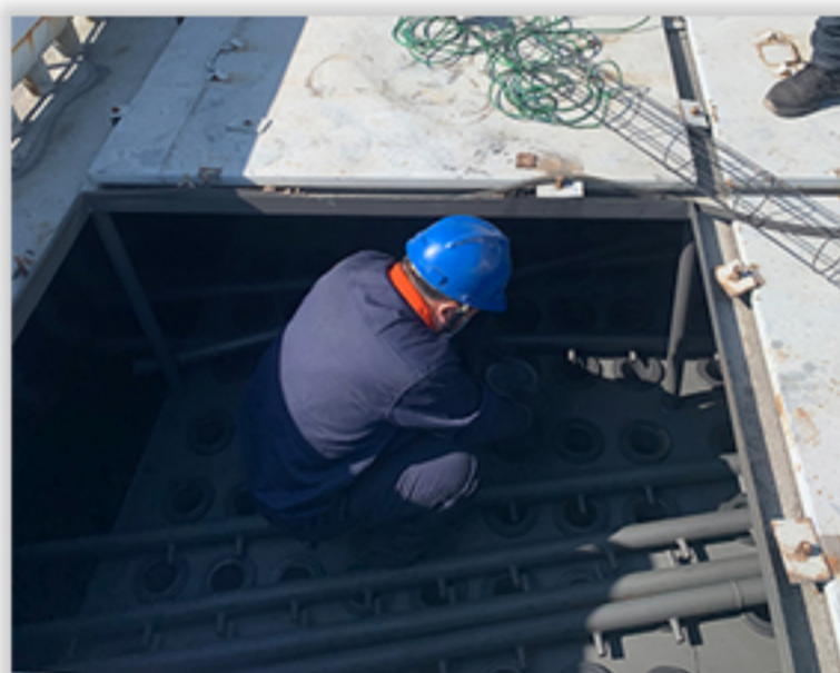
repair dust collector in steel plant project
